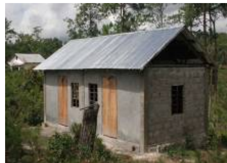
New school building in Kut
